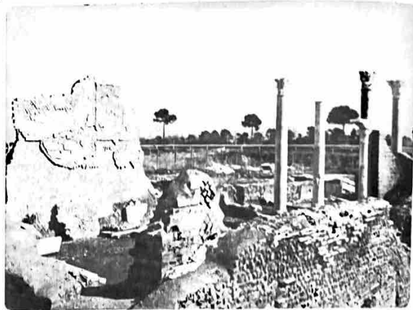
FIG. 12 THE MAIN HALL OF THE SYNAGOGUE AFTER RESTORATION—FROM THE WEST. THIS LINKS WITH THE VIEW SEEN IN FIG. 3.
