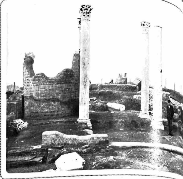
FIG. 6. AFTER THE RE-ERECTION OF THE FOUR CORINTHIAN COLUMNS WHICH FORMED THE MONUMENTAL ENTRANCE TO THE MAIN HALL.
