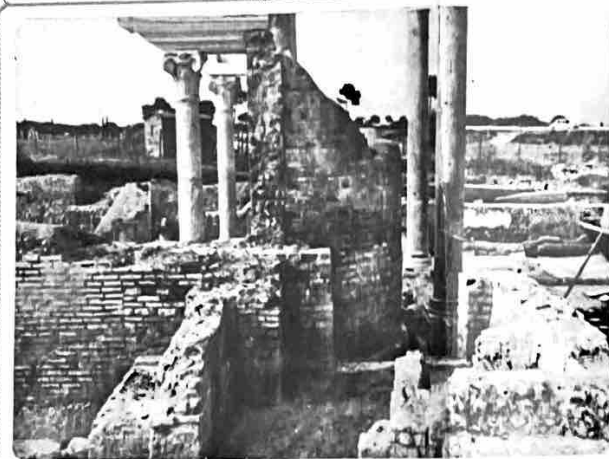
FIG. 11 THE LITTLE CORRIDOR, LEADING FROM THE MAIN HALL (BACKGROUND) TO THE MEETING ROOM (LEFT FOREGROUND). (SEE FIG. 8.)
