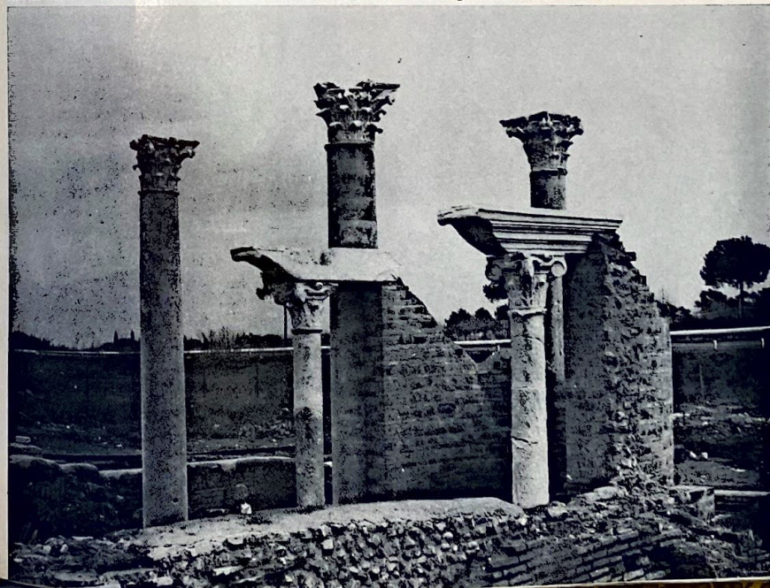
Closer view of the aedicula with its colonnettes and architraves ending in corbels.
