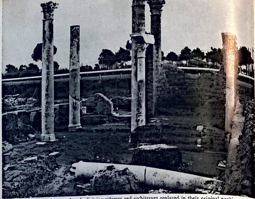
The aedicula of the Torah restored, and adjoining columns and architraves replaced in their original position.
